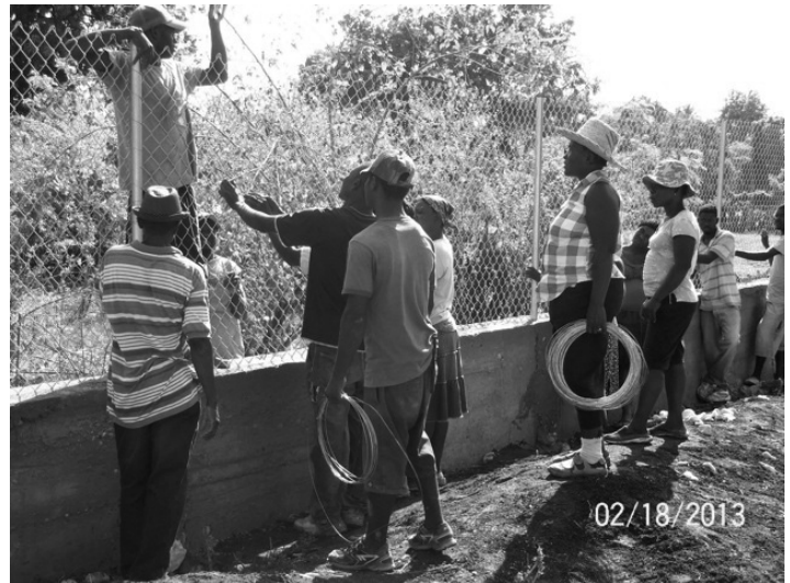
Installing the perimeter wall.
