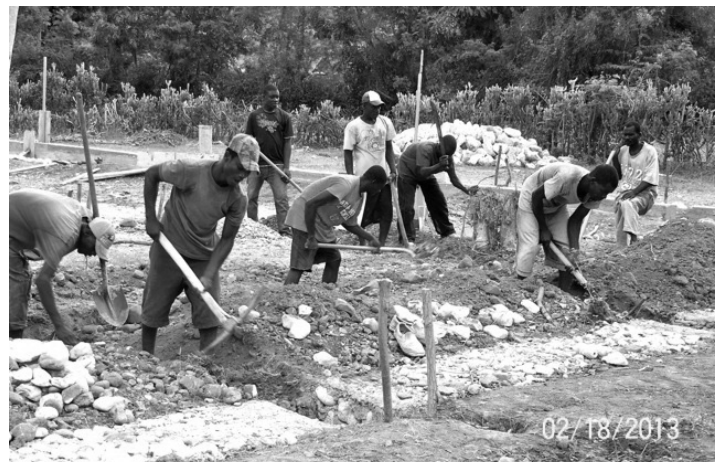
Working on the foundation for guard house wall.
