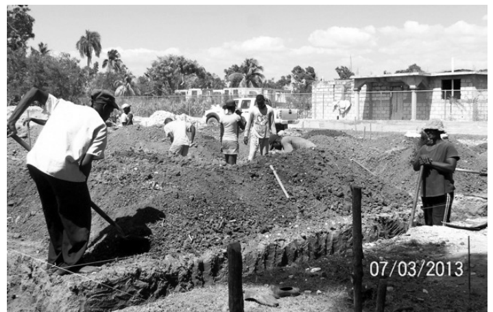
Staking and digging the library foundation wall.
