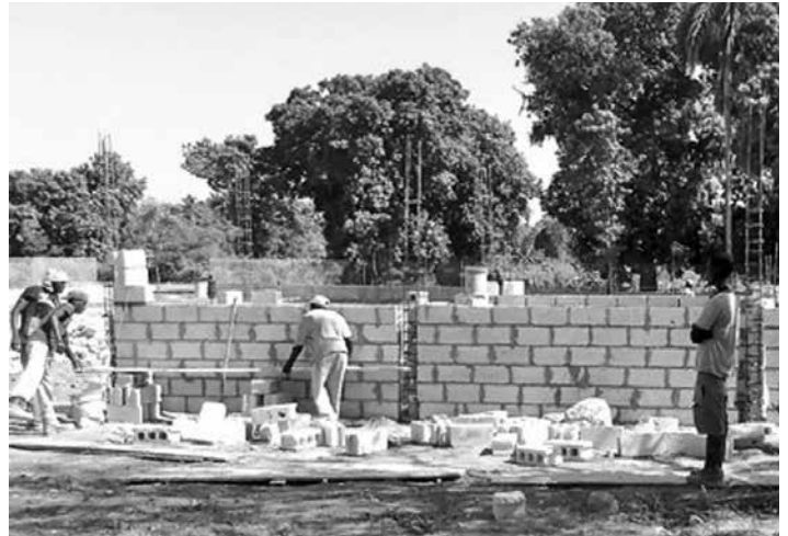
Guardhouse, pump house, depot.
